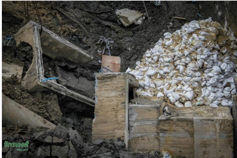
Sealing the tunnel by sandbag
